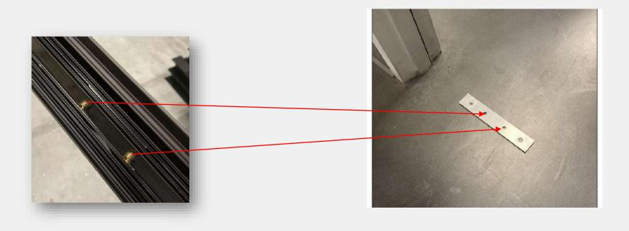
NOTE: Apply ample amount of silicone under the sill as part of installation.
