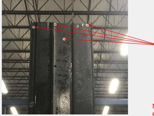
Apply a strip of silicone between the Jamb and the Head
